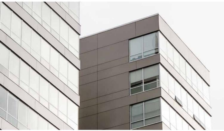
"The Trespa<sup>®</sup> cladding panels did a great job of seamlessly unifying the appearance of the renovated existing building with the new building expansion, more than doubling the original building's size."
